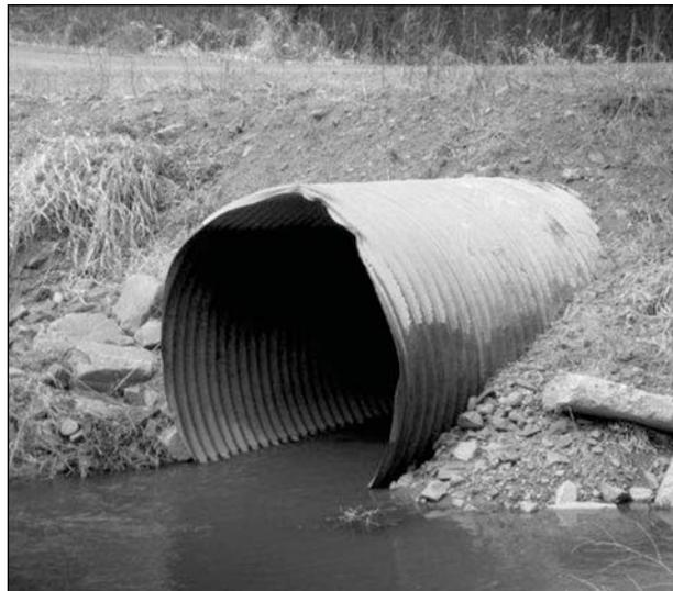
*This problem culvert is on Mattson Road at an unnamed tributary to the Marengo River in the Town of Ashland. It is currently an erosion problem and at risk of failure, and is slated to be replaced in 2012.*
